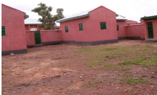
Fig. 3 New Settlement at Maiganga
