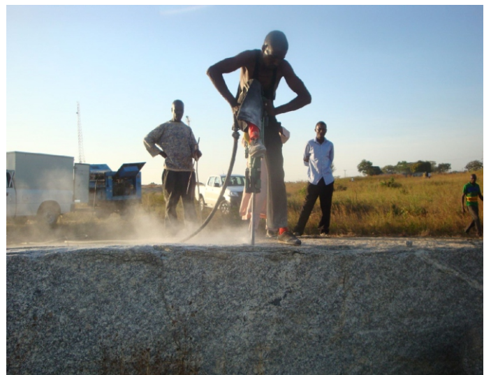
Fig 3 : Drilling process going on using jack hammer drilling machine
