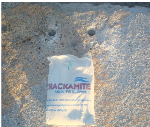
Fig. 4: Expansive chemical and the drilled holes in preparation for mixing
