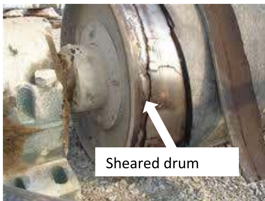
Figure 4: Damaged bearing and pulleys due to torsional stress
